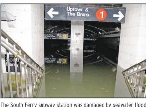
The South Ferry subway station was damaged by seawater flooding during Hurricane Sandy. Photo courtesy Leonard Wiggins/MTA
