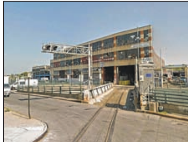
The Federal Railroad Administration is looking into traffic signal issues at a Maspeth crossing.
