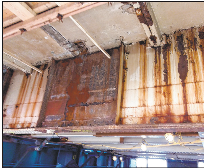
The steel beam holding up the western platform of the N/W 36th Avenue station in Astoria is rusted through in many places.
