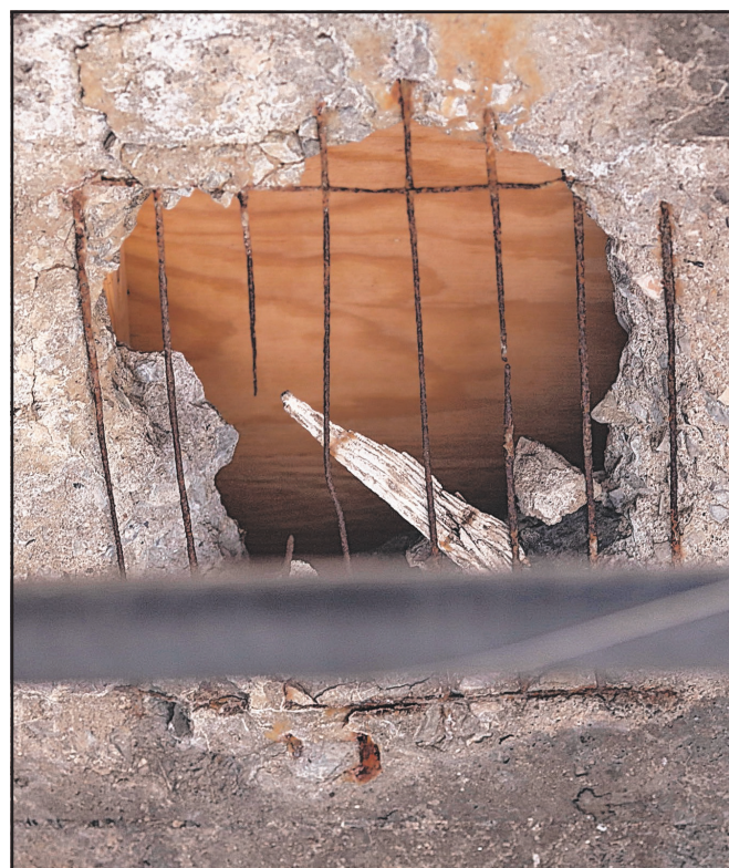
The floor under the health food store on the bridge is starting to rot. This is the view from the station platform looking up.
